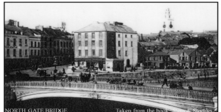
NORTH GATE BRIDGE
