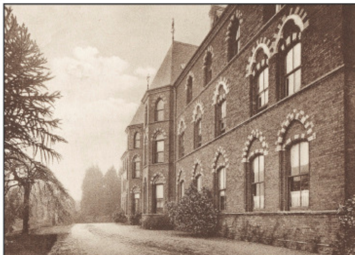
Eastern view of Farranferris College, Cork Photo: Courtesy of St Finbarr's College, Farranferris
