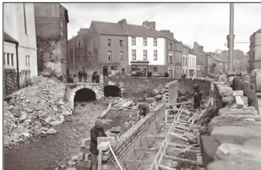
Road widening at Blackpool Bridge, Cork, 1953 site of the Roaring Bridge Photo: Courtesy of The Irish Examiner Ref. 932E
