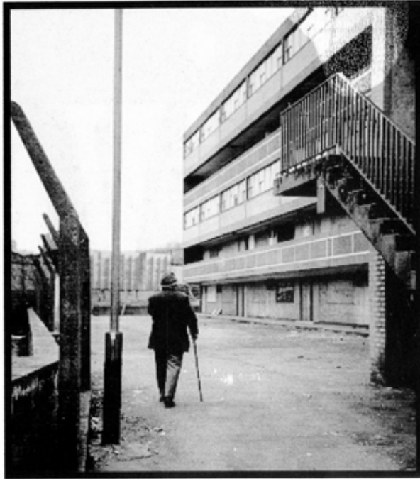
The site of Bird's Quay
